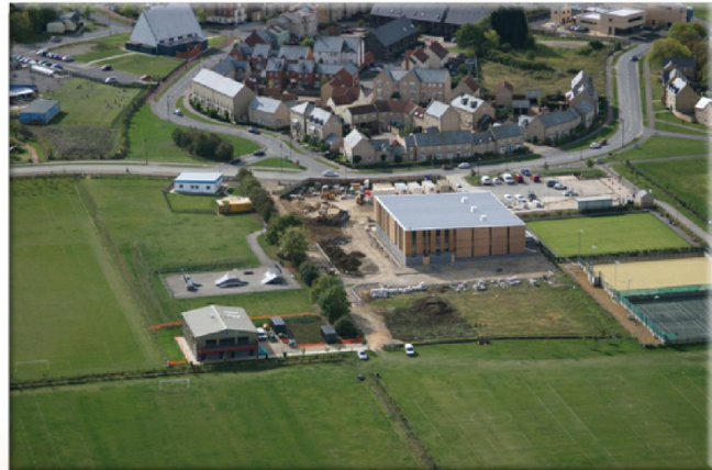
Above: Aerial view of Sports Centre construction site
